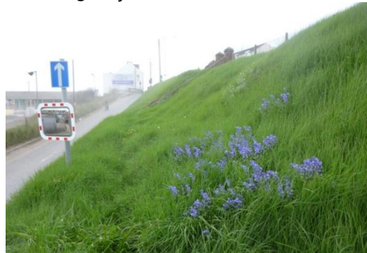
Basin Road North embankment
